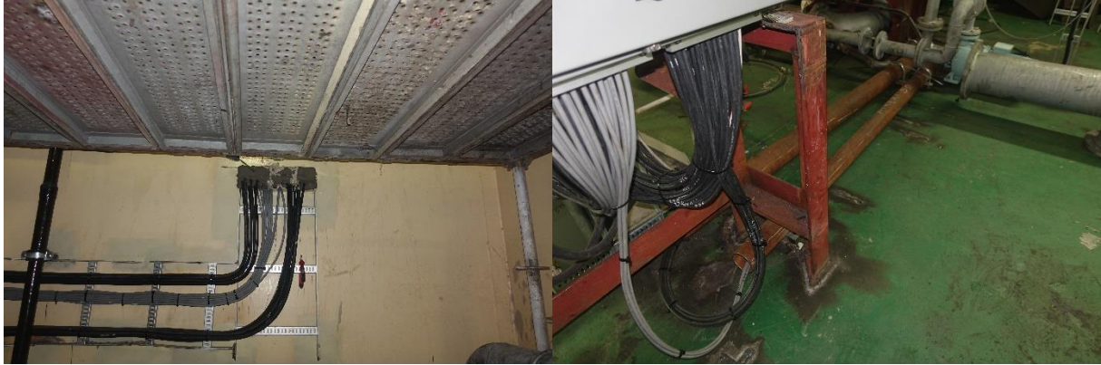
Figure 225 – Bulkhead Penetration & Cabling of BWTS Components to Electric Panel
