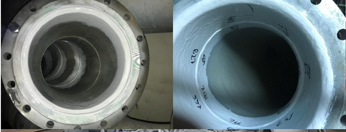
Figure 135 - Repairing (Coating) of Galvanized Pipes with RL 500PF + RA 500M Glassflake
