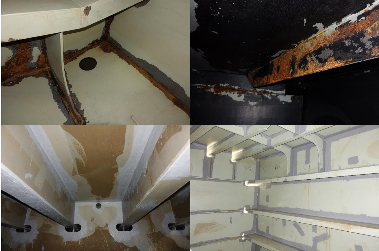
Figure 180 - Waterjetting & Spot Coating Application for Ballast Tanks
