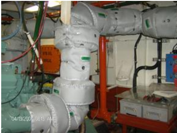
Figure 133 - Pipe Insulation Jackets
