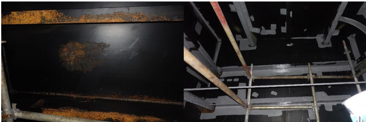
Figure 59 - Ballast Tank TU Coating Application with RS 500P – Sefine Shipyard
