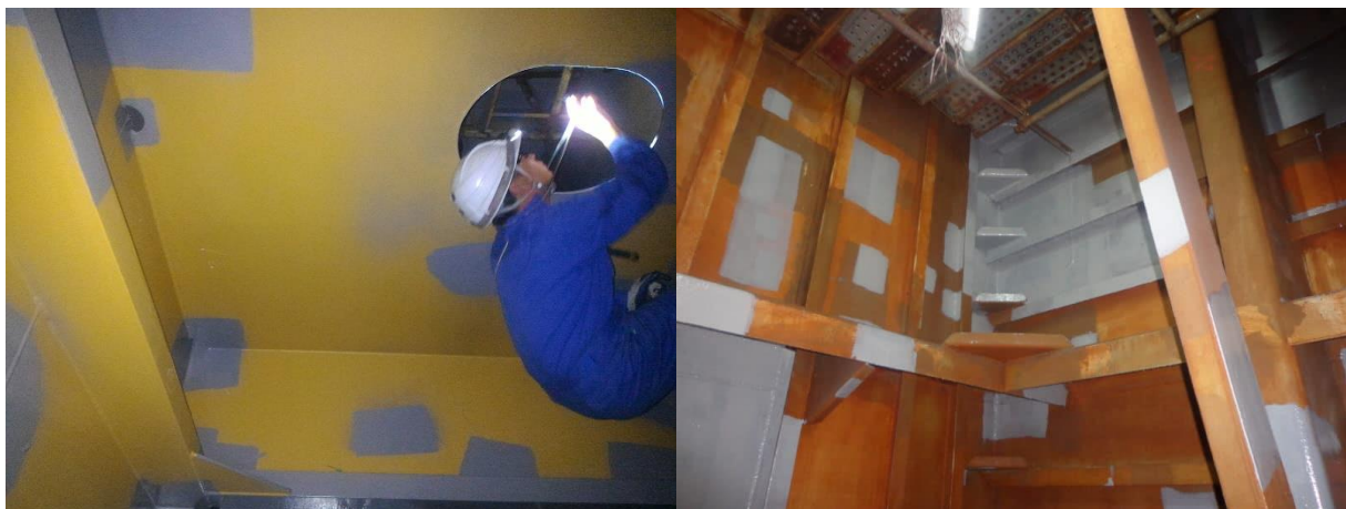
Figure 187 - Fresh Water Tank Patch Repairs (RS 500P + RA 500M Solvent Free Epoxy)
