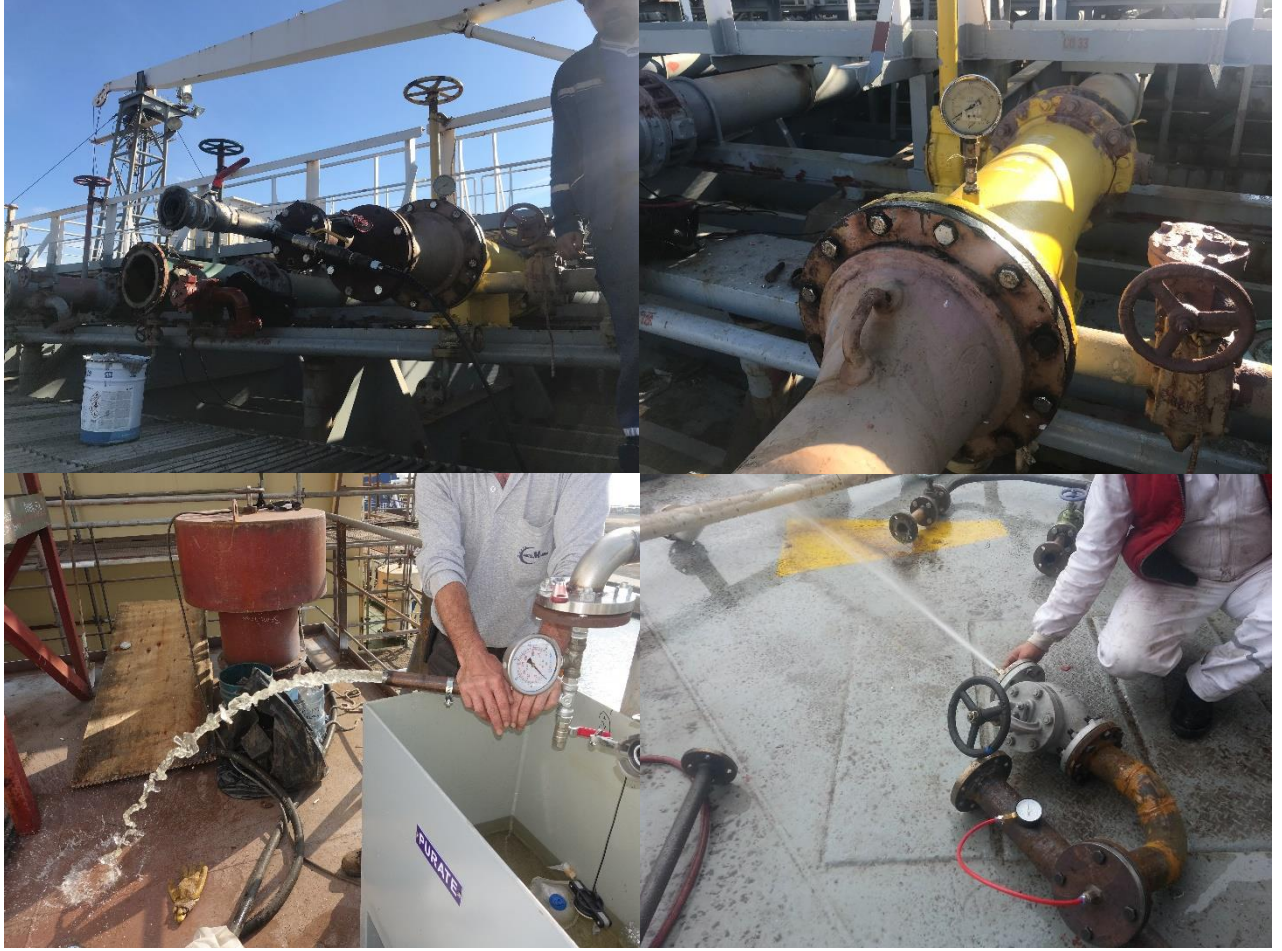
Figure 123 - Pressure Testing of Lines (Hydrostatic Tests)
