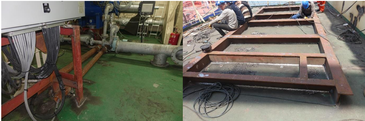
Figure 110 - Panel and Chemical Tank Foundations
