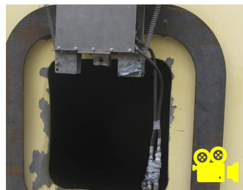
Figure 92 - Cold Cutting with Waterjets (Exproof) on Hull
