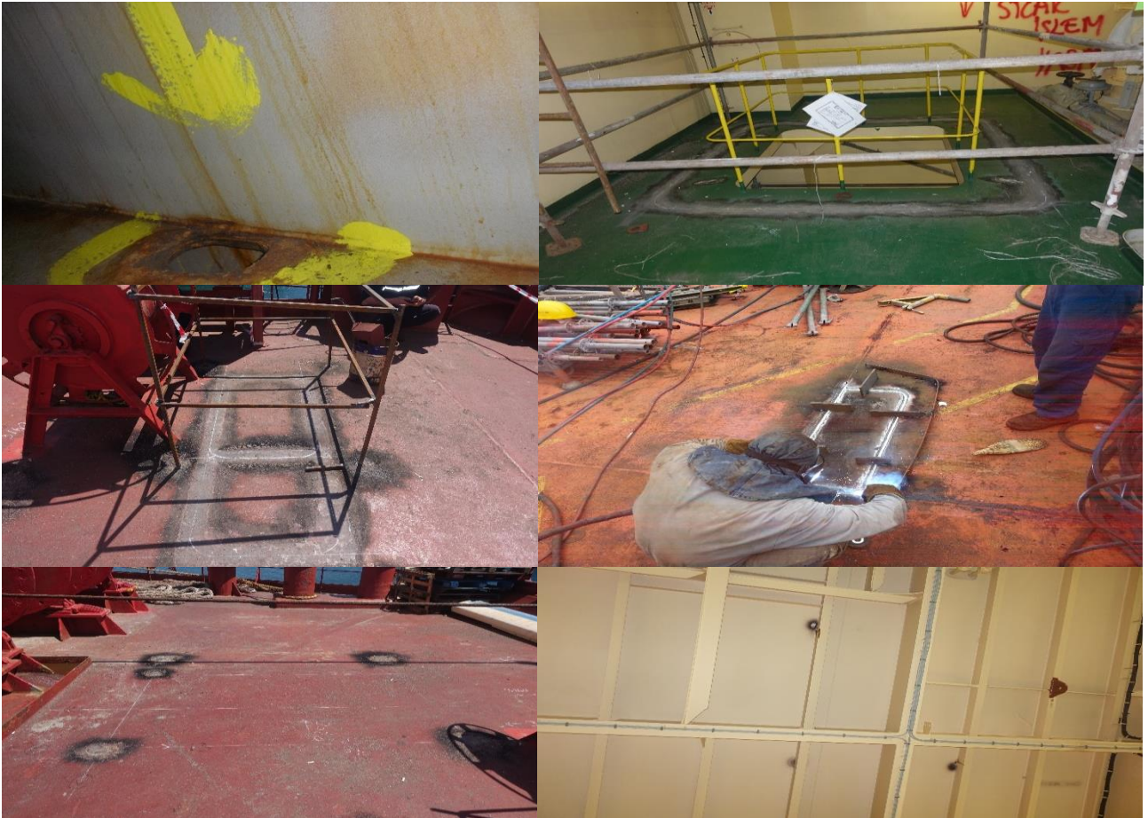
Figure 87 - Marking of Steel Plates Before Cropping
