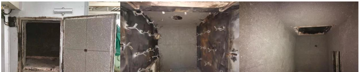
Figure 199 - Refractory Application Process
