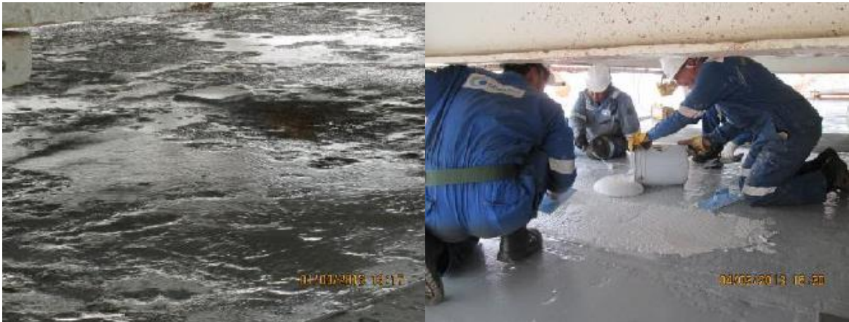
Figure 100 - Epoxy Repairs on Pittings (Offshore or Accommodation Decks)
