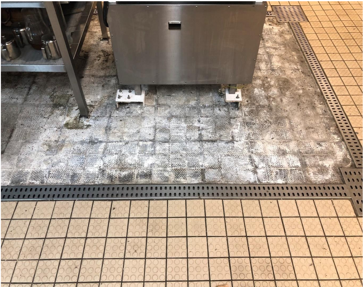
Figure 209 - Galley Floor Needs Epoxy Coating Repair
