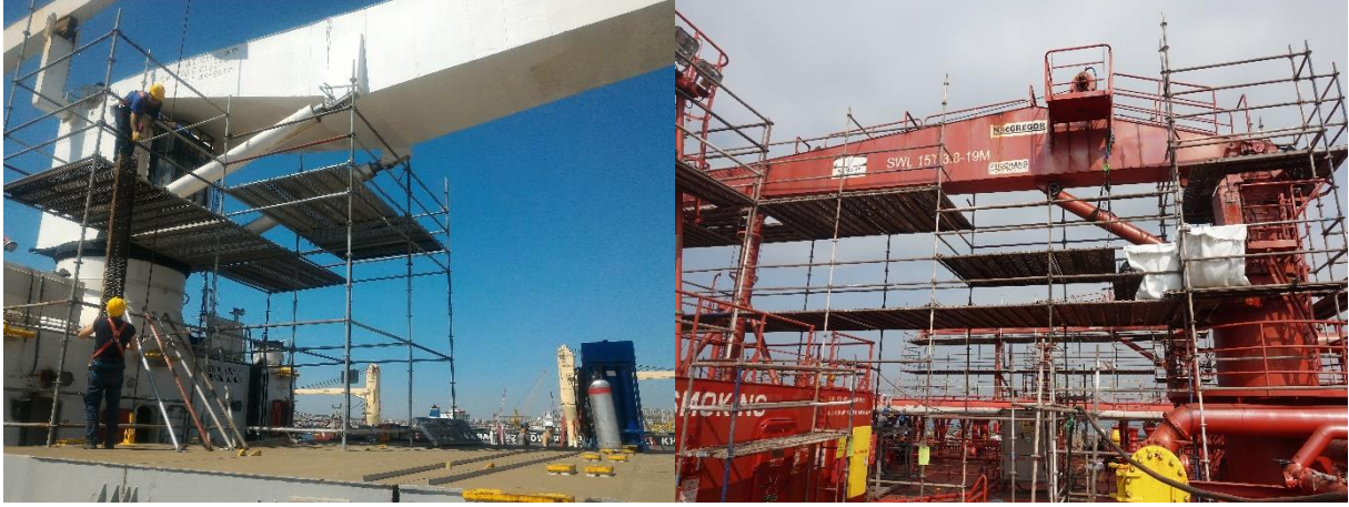
Figure 72 - Crane Hydraulic Piston Repairs with Safe Staging
