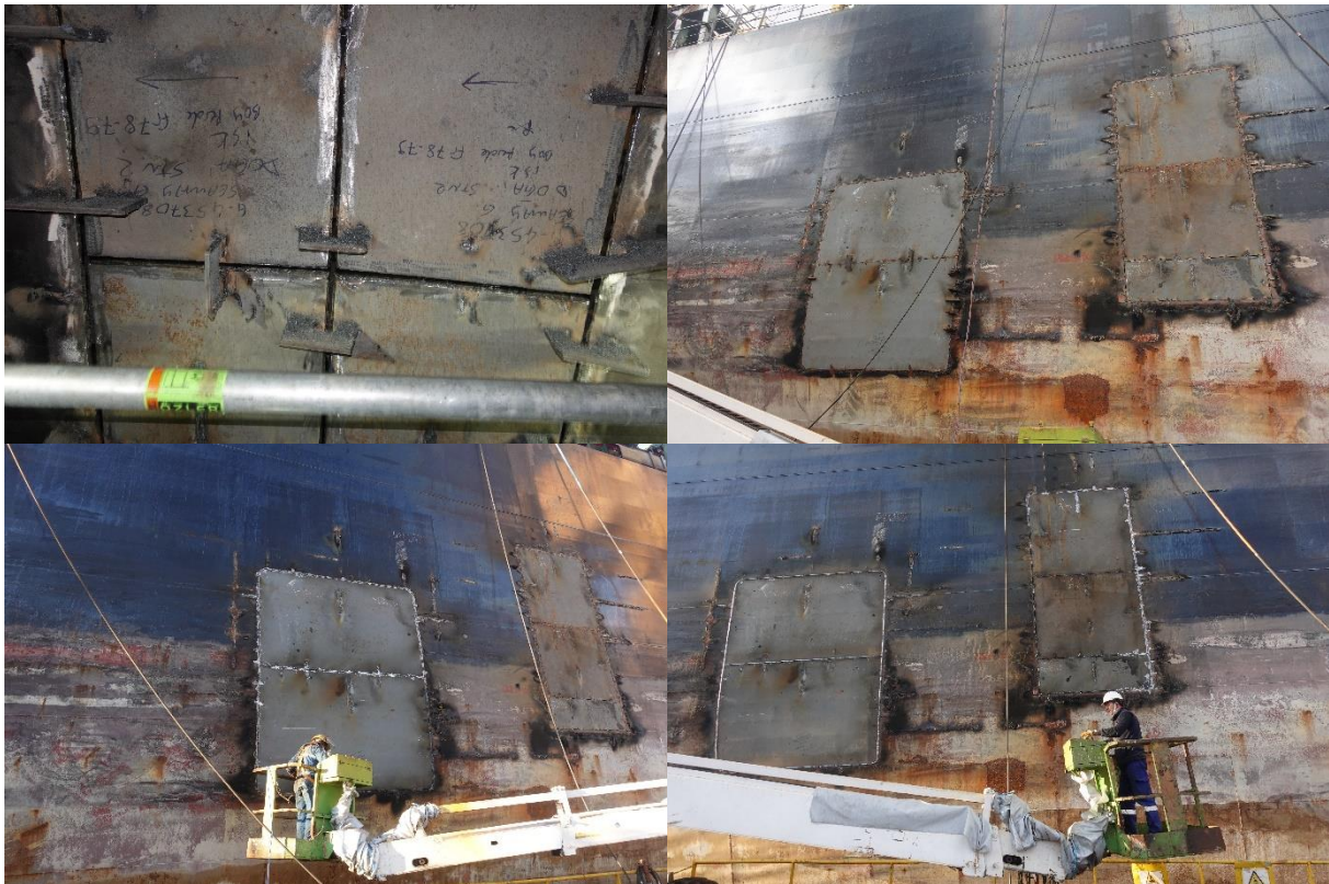
Figure 91 - Steel Renewal on Hull & Cargo Bulkheads
