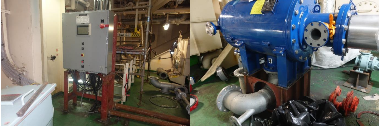
Figure 220 - Electric Panel and Filter Foundations
