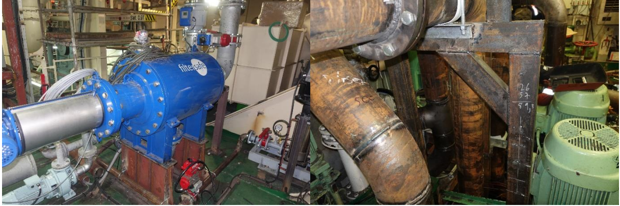
Figure 109 - BWTs Equipment and Pipe Foundations - Supports
