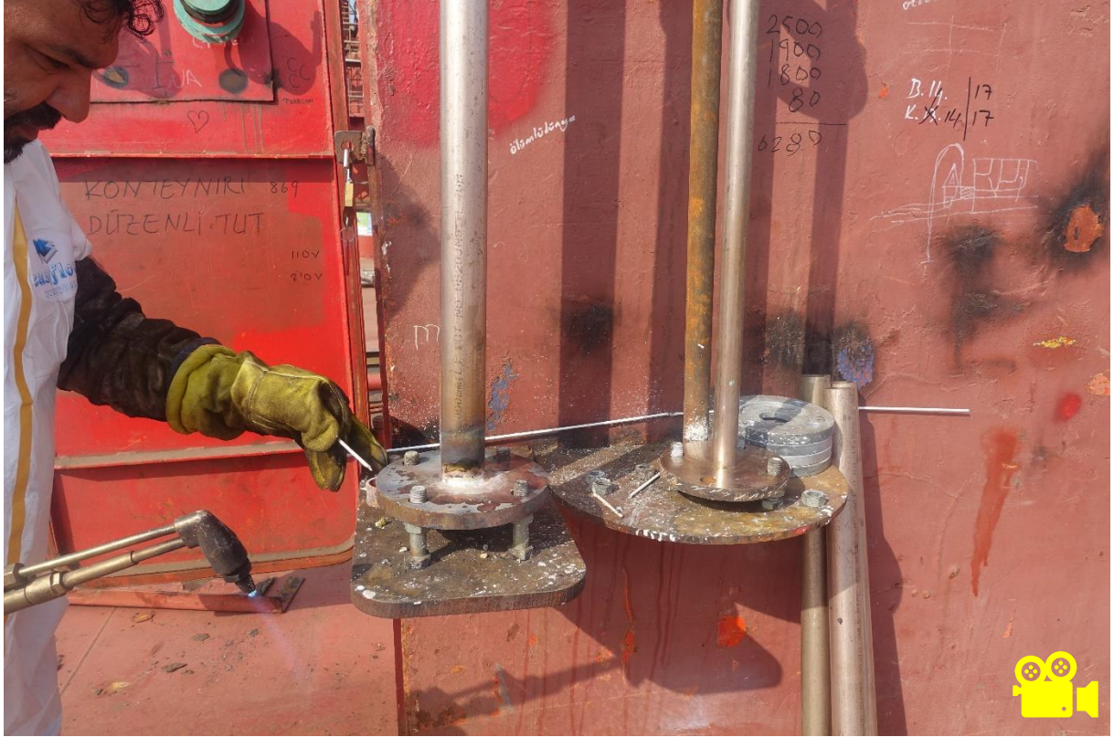
Figure 127 - Heating Coil Welding
