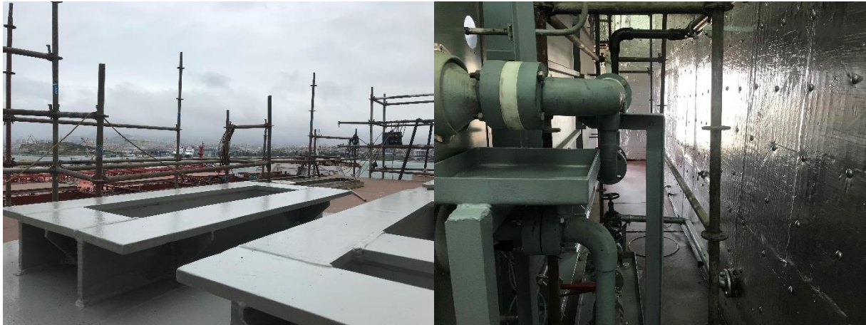
Figure 216 - BWTs Chemical Tank Foundation and Drip Tray Under the Flanges – TK Tuzla Shipyard
