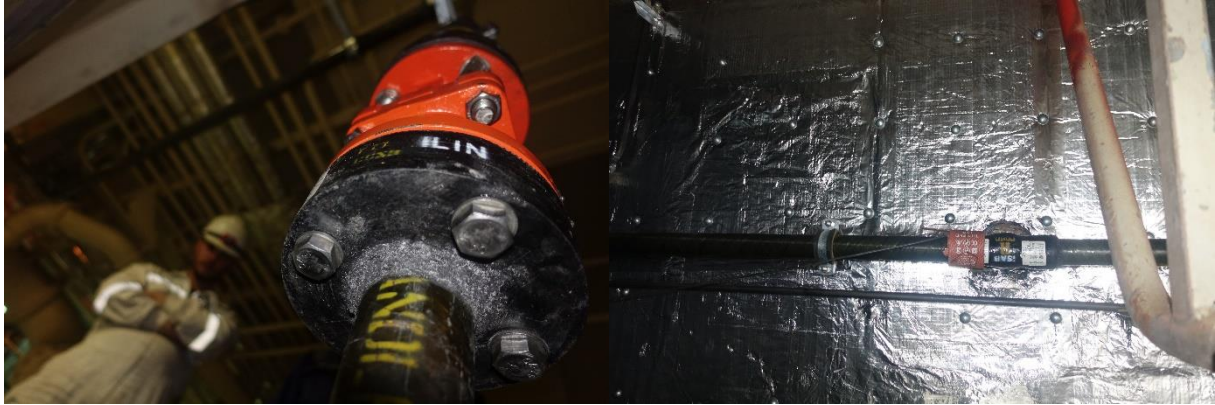
Figure 131 - GRE Pipe Heat Curing Process
