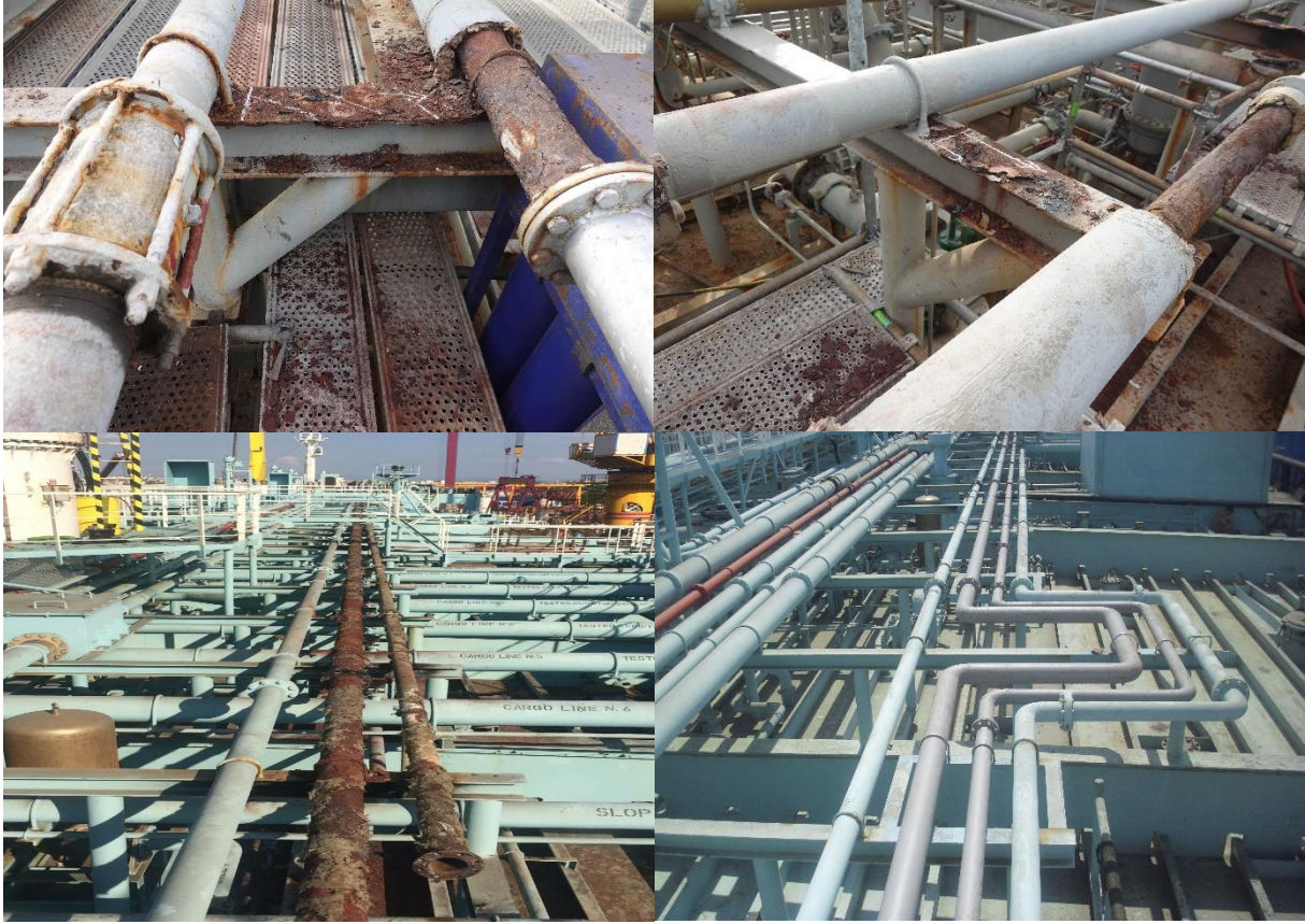
Figure 138 - Corrosion Under the Insulation and Coating Protection with Chemco RL 500PF
