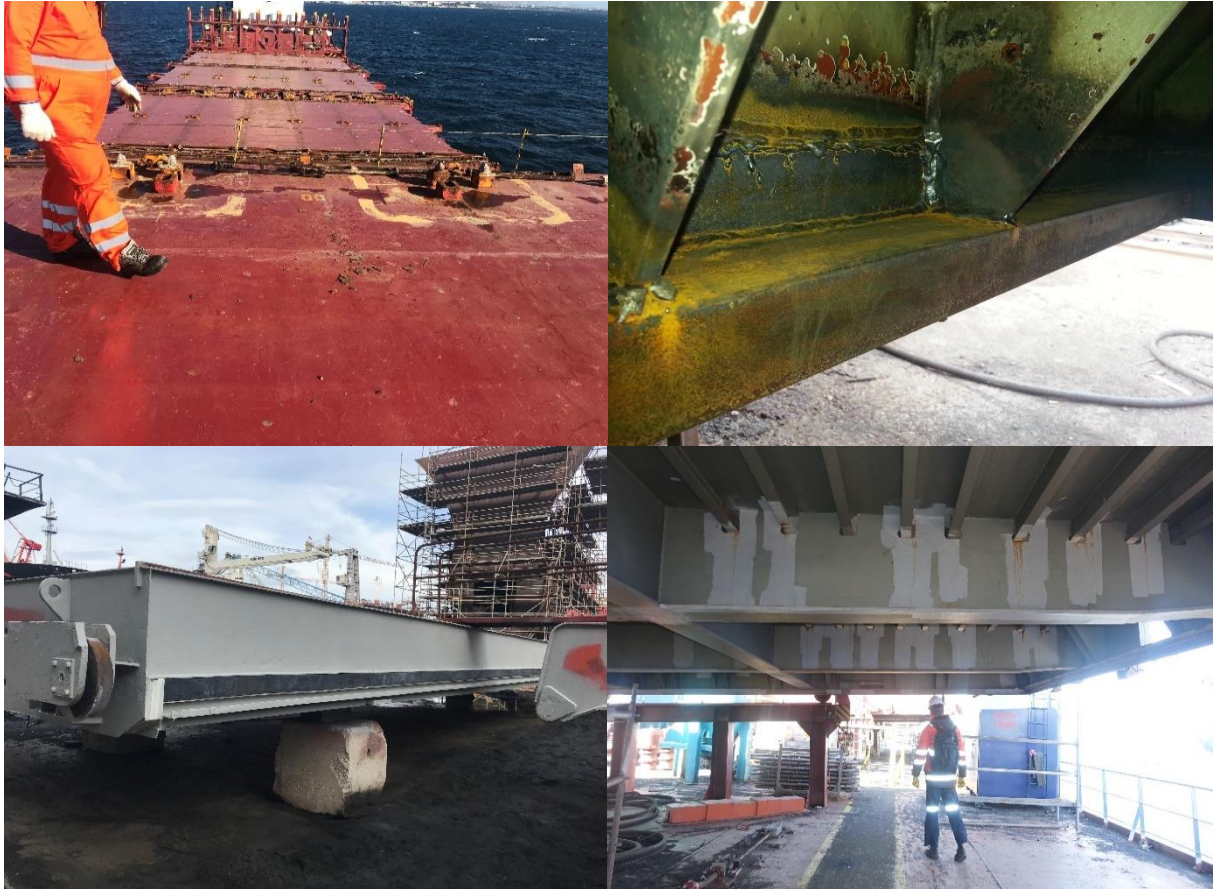
Figure 115 - Hatch Cover Steel & Coating Works
