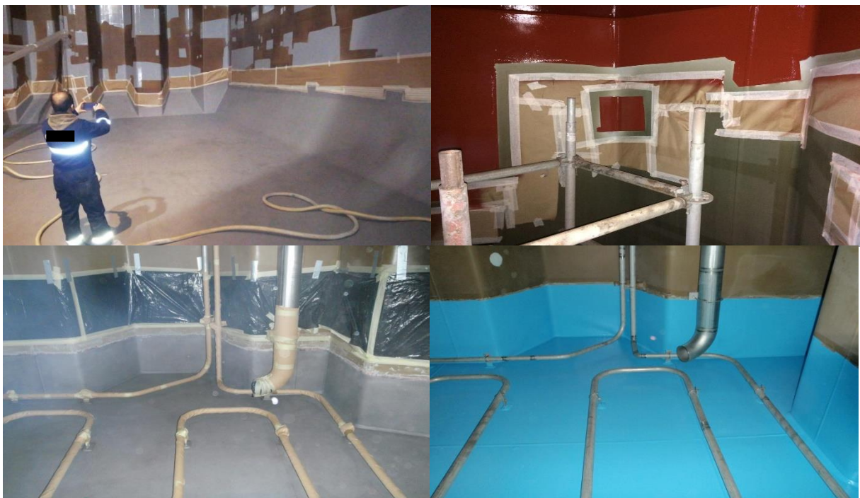
Figure 185 - Cargo Tank Coating Repairs
