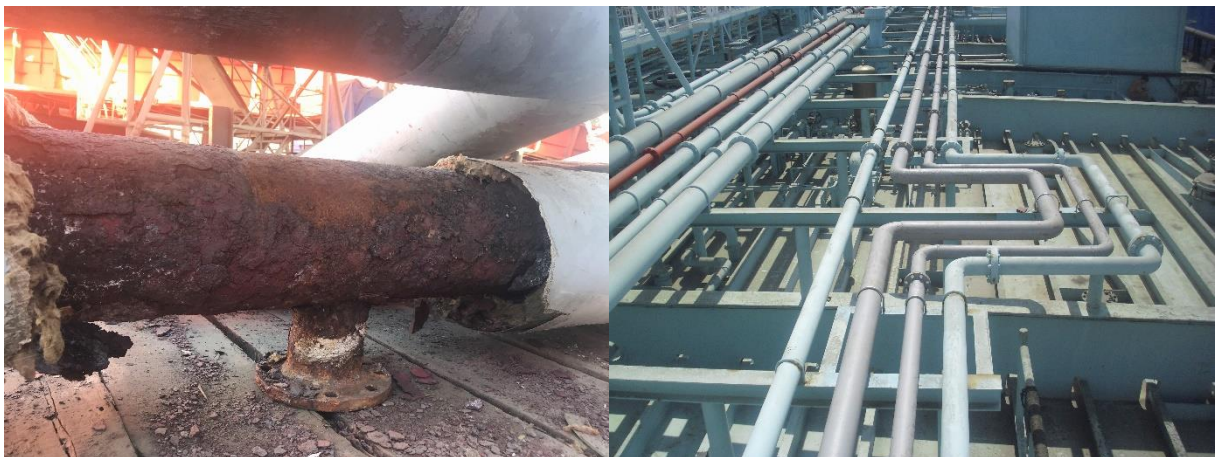
Figure 188 - Steam Line Corrosion (CUI) and Coating Application (RL 500PF)
