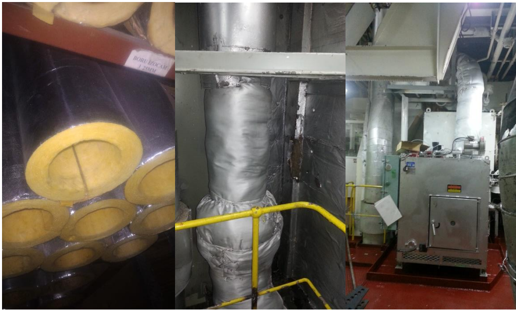
Figure 205 - Pipe Insulation Applications
