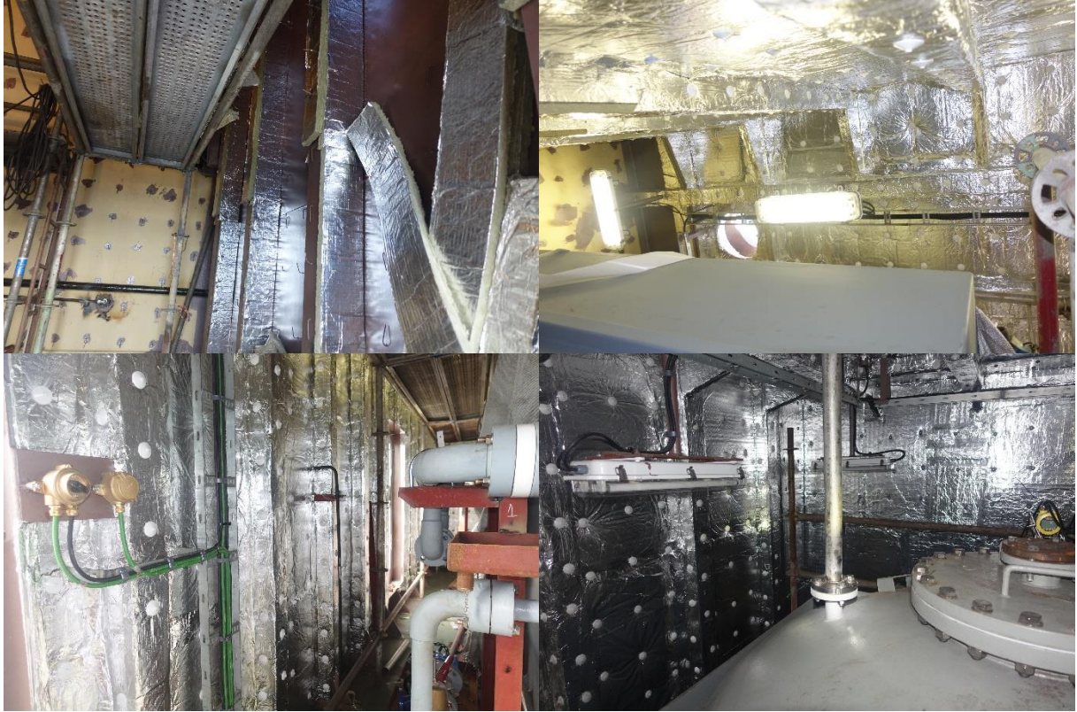
Figure 204 - Insulation for Rooms & Bulkheads
