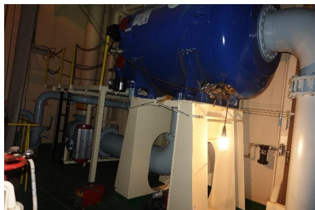
Figure 214 - BWTS Filter Foundation
