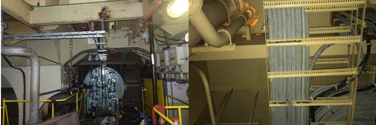
Figure 111 - Cable Trays
