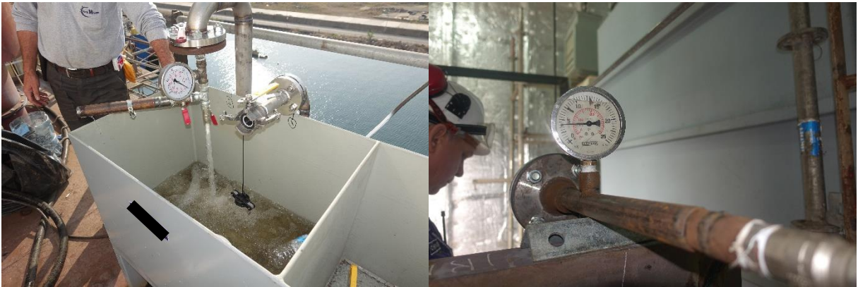
Figure 224 - Pressure Testing of Lines Before Commissioning
