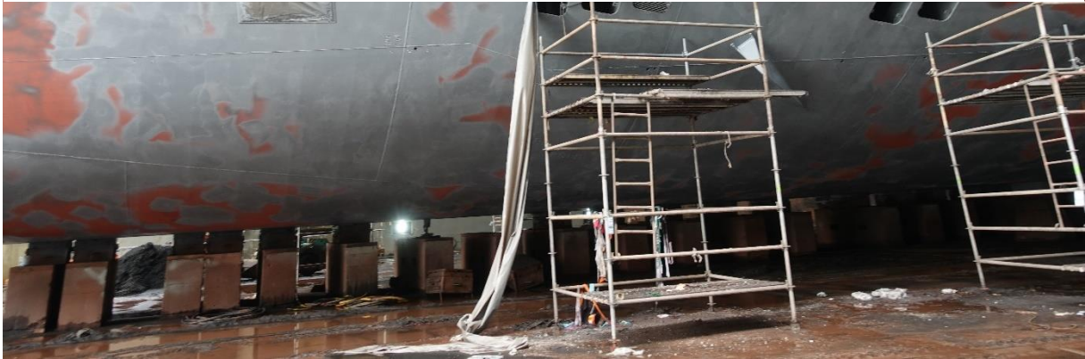
Figure 41 - ICCP Protection During the Hull Coating & Seachest Coating
