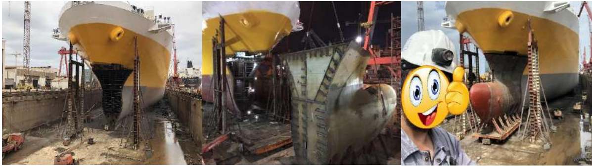
Figure 170 - Bulb Modification (Besiktas Shipyard)
