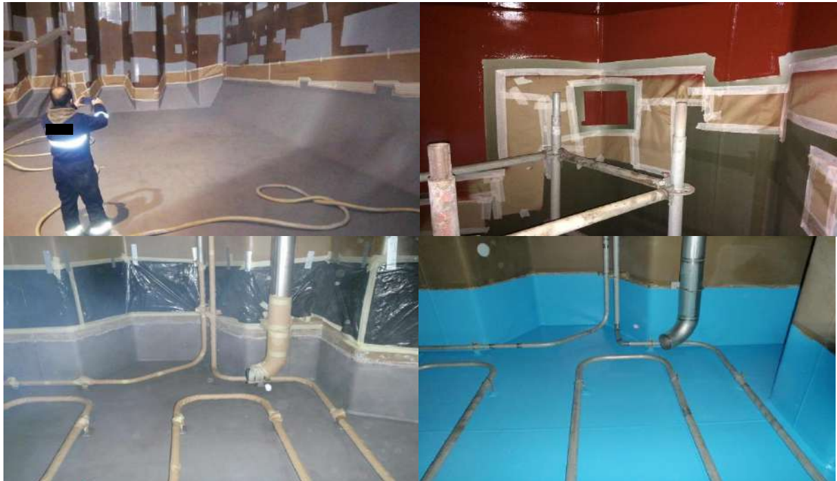
Figure 185 - Cargo Tank Coating Repairs
