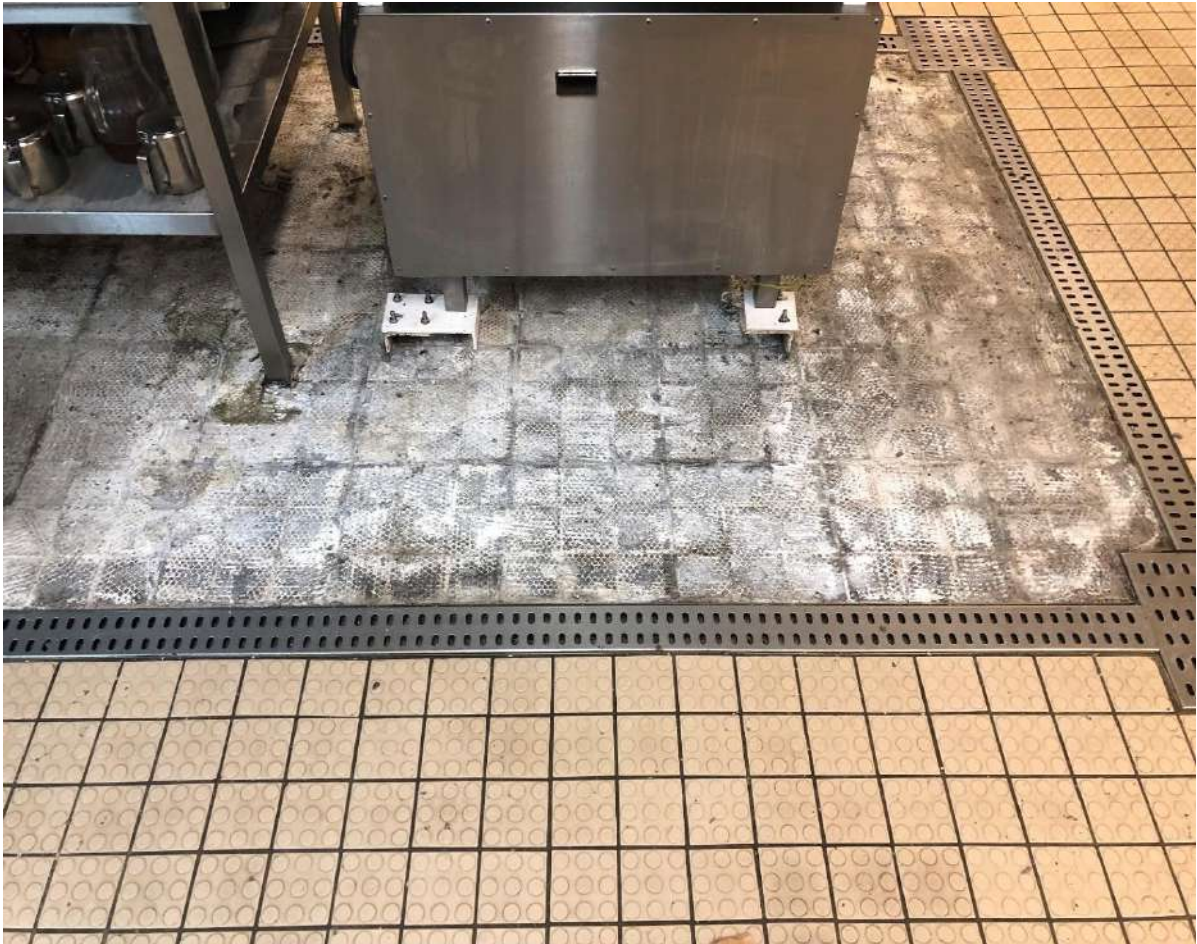
Figure 210 - Galley Floor Needs Epoxy Coating Repair
