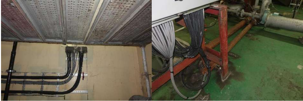
Figure 226 – Bulkhead Penetration & Cabling of BWTS Components to Electric Panel
