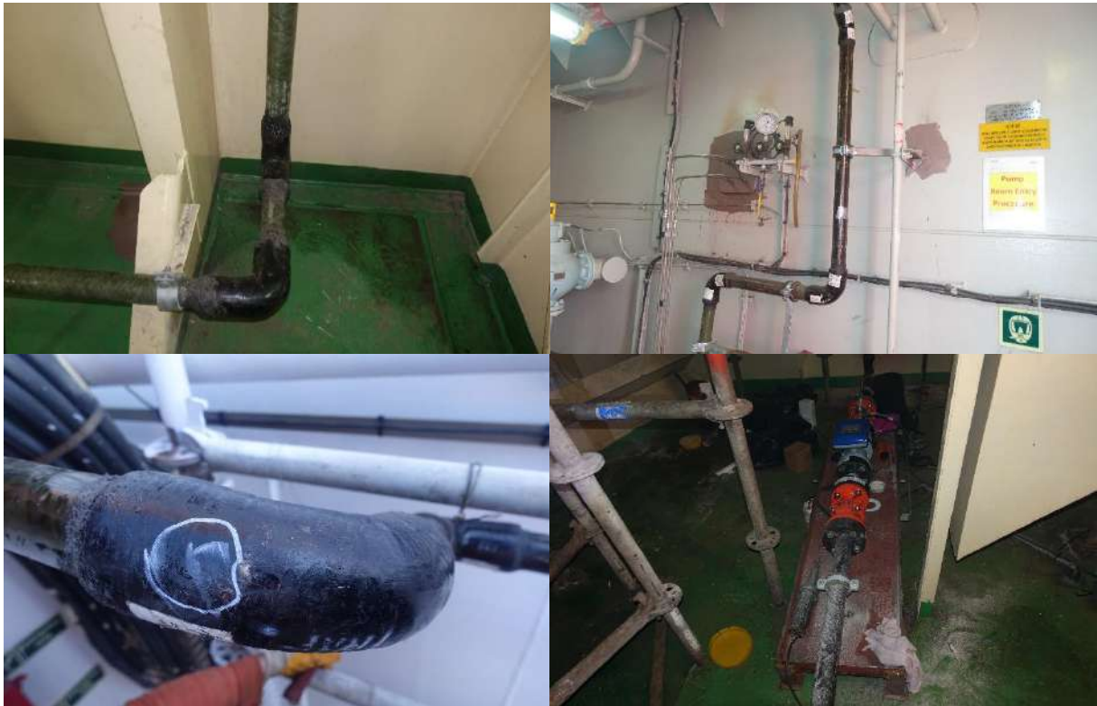
Figure 130 - GRE & GRP Pipe Fabrication and Inspections
