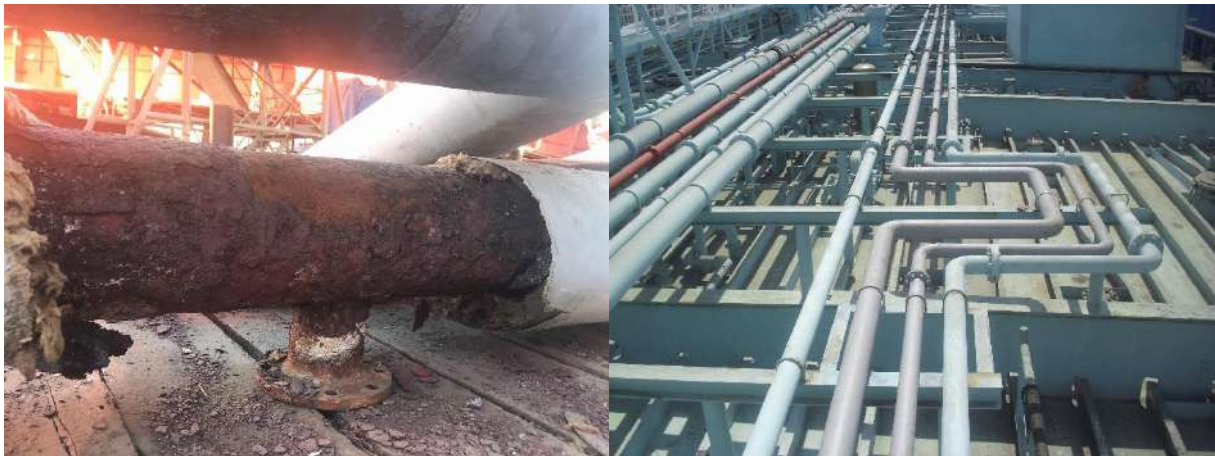
Figure 189 - Steam Line Corrosion (CUI) and Coating Application (RL 500PF)
