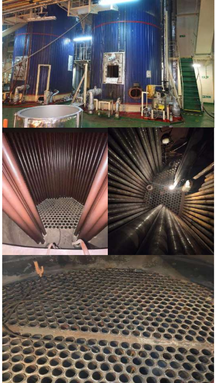
Figure 198 - Boiler Pipe Renewal Works
