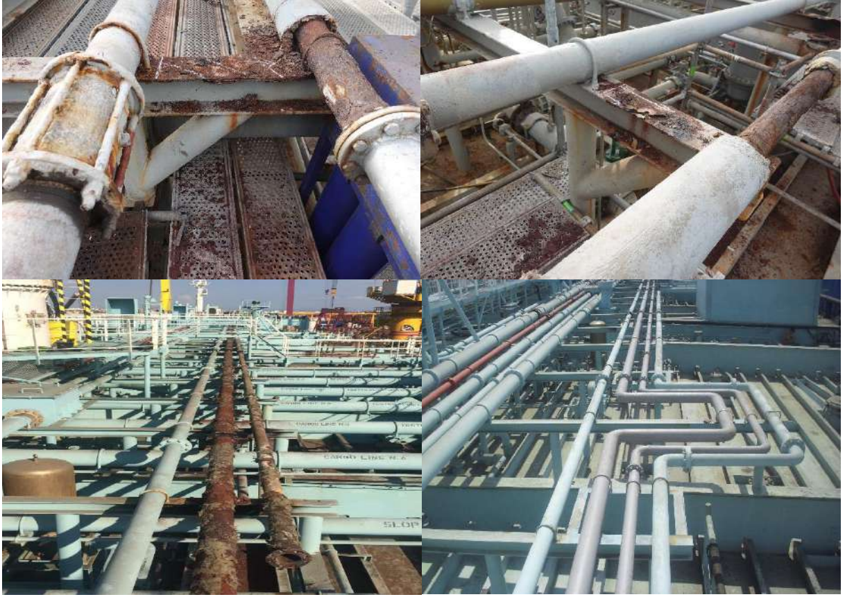
Figure 139 - Corrosion Under the Insulation and Coating Protection with Chemco RL 500PF
