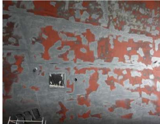
Figure 55 - ICCP Protection
