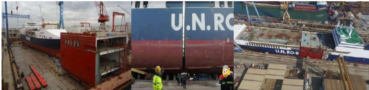
Figure 172 - Ship Lengthening (Gemak Shipyard - 30 meter)
