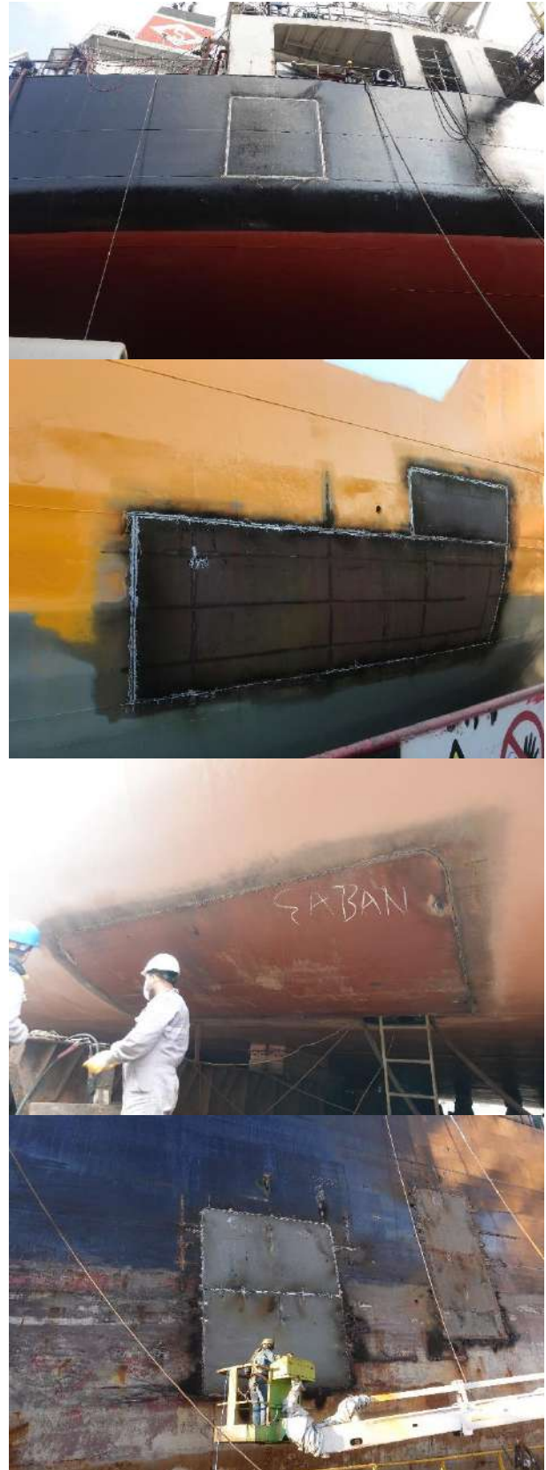
Figure 43 - Hull Steel Inserts
