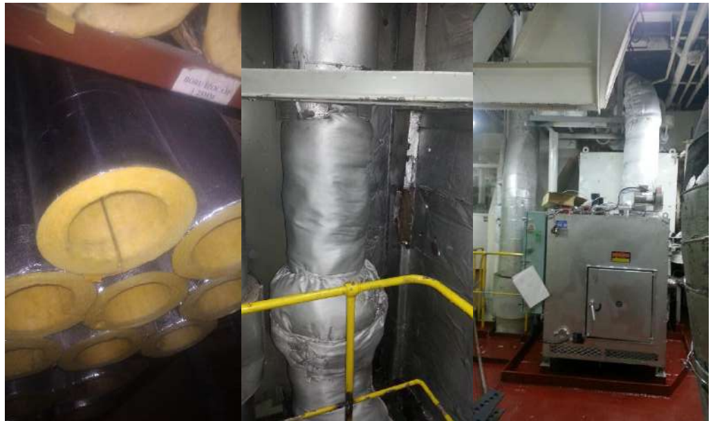
Figure 206 - Pipe Insulation Applications
