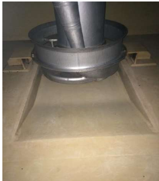
Figure 196 - Cargo Pump Bellmouth Suction
