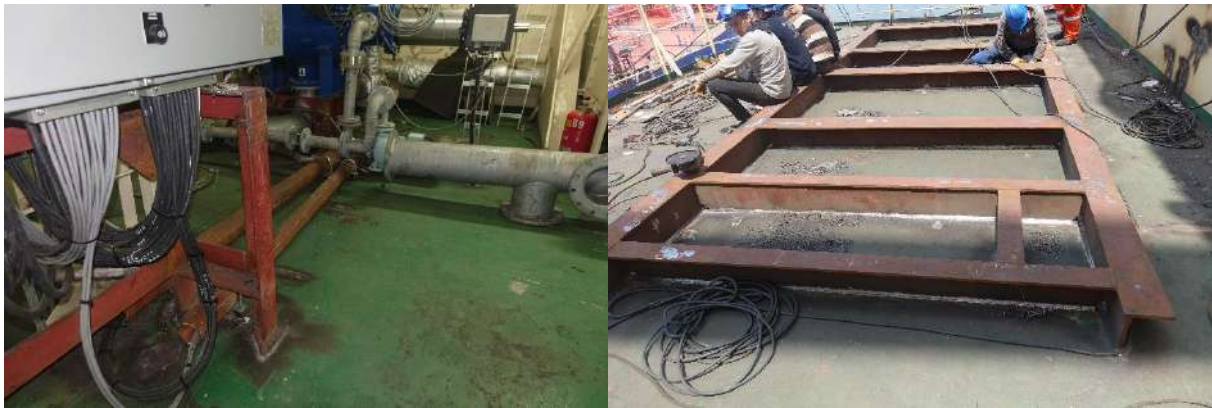
Figure 110 - Panel and Chemical Tank Foundations
