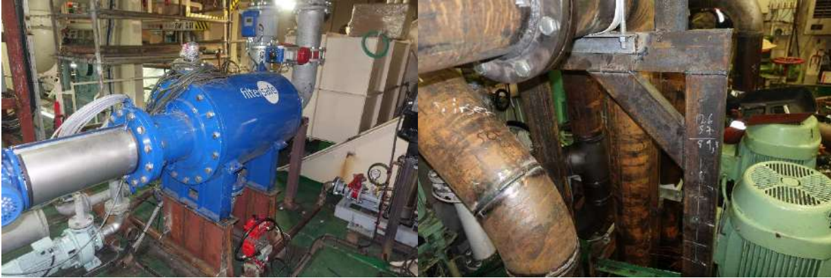
Figure 109 - BWTS Equipment and Pipe Foundations - Supports
