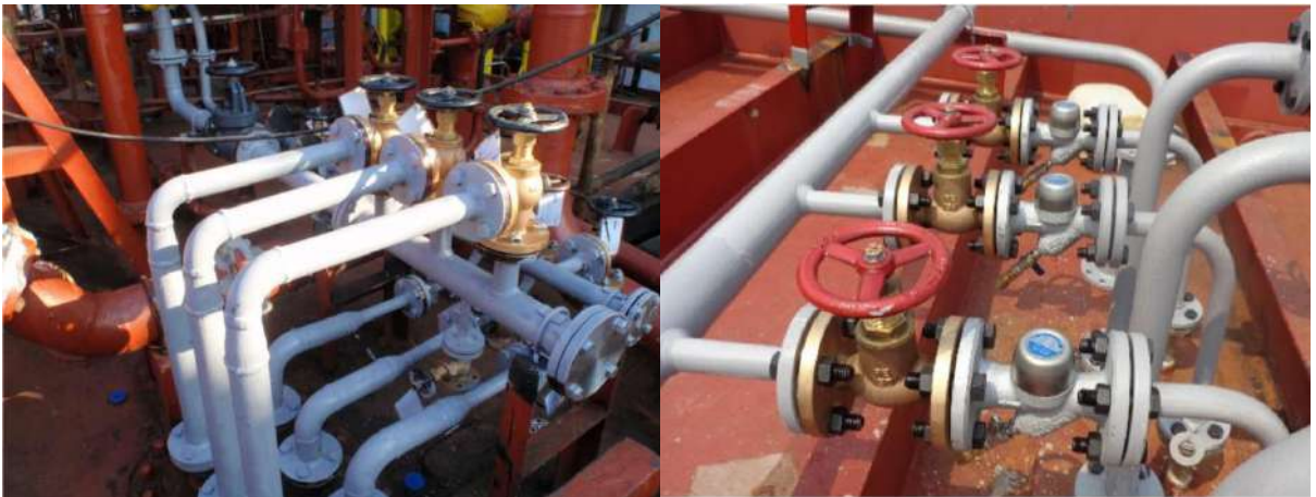
Figure 138 - Chemco RL 500PF Application on Heated Lines
