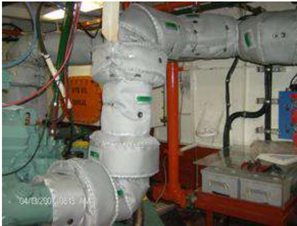
Figure 133 - Pipe Insulation Jackets
