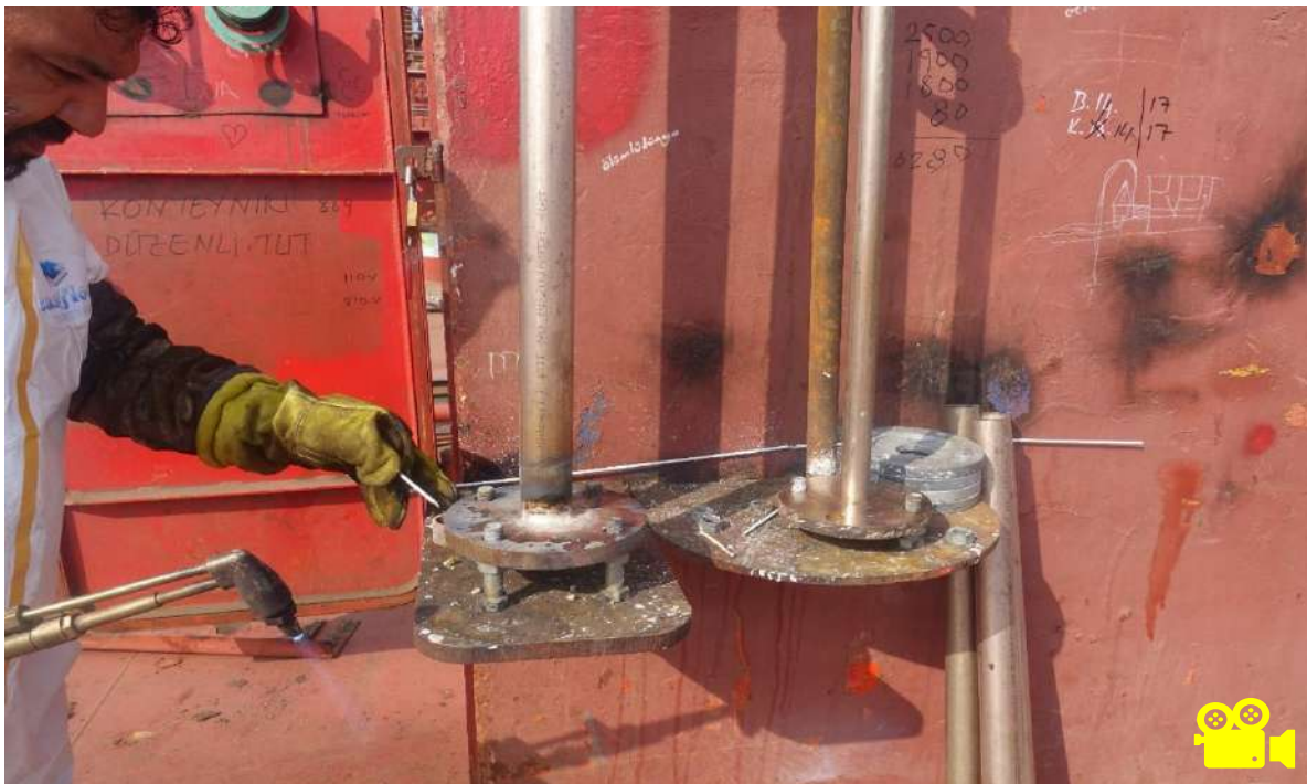
Figure 127 - Heating Coil Welding
