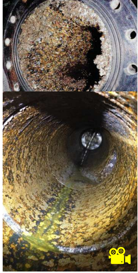
Figure 126 - Pipe Internal Cleaning and Coating Application via Robots
