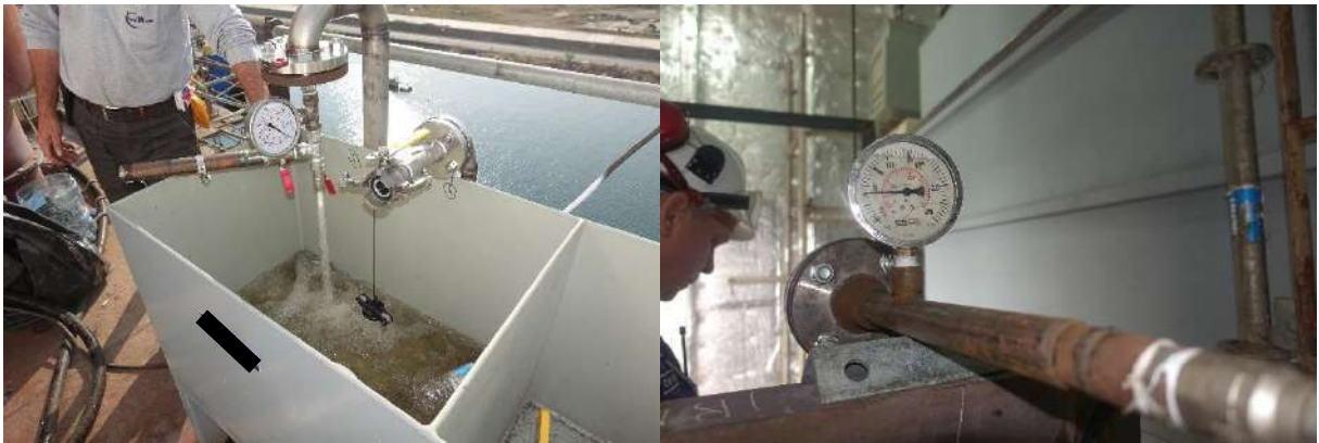
Figure 225 - Pressure Testing of Lines Before Commissioning
