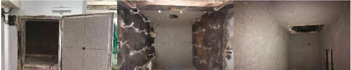
Figure 200 - Refractory Application Process
