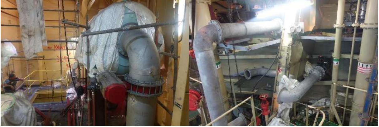
Figure 224 - BWTS Line Installations
