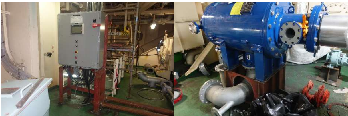
Figure 221 - Electric Panel and Filter Foundations
