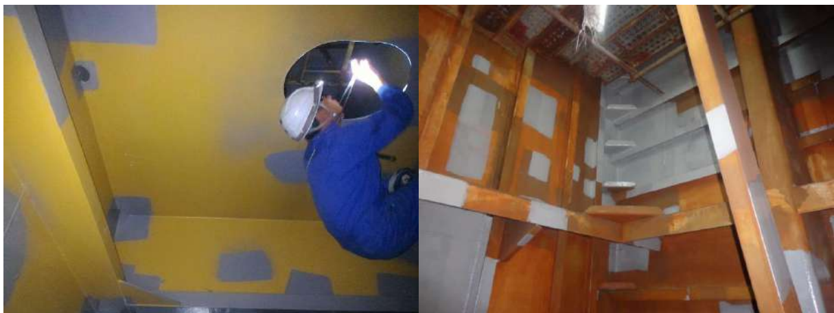
Figure 188 - Fresh Water Tank Patch Repairs (RS 500P + RA 500M Solvent Free Epoxy)
