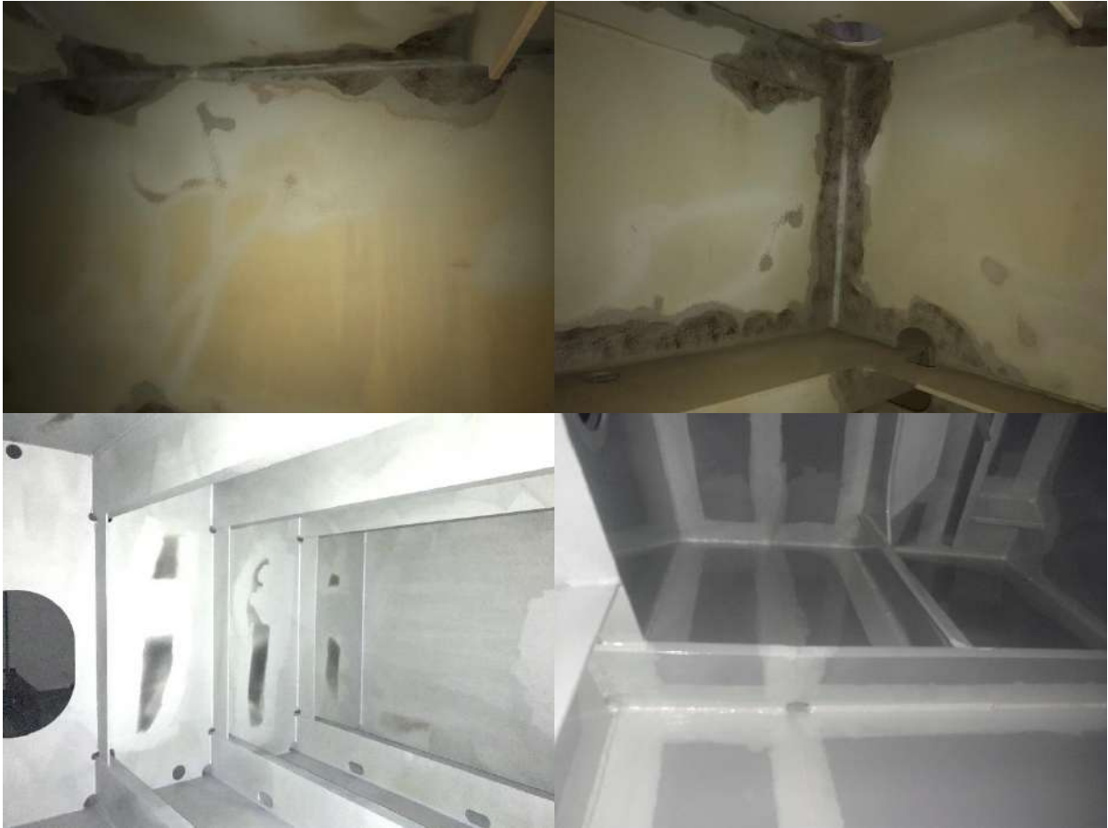
Figure 179 - Blasting of Ballast Tanks and Coating Application (Traditional Epoxies)
