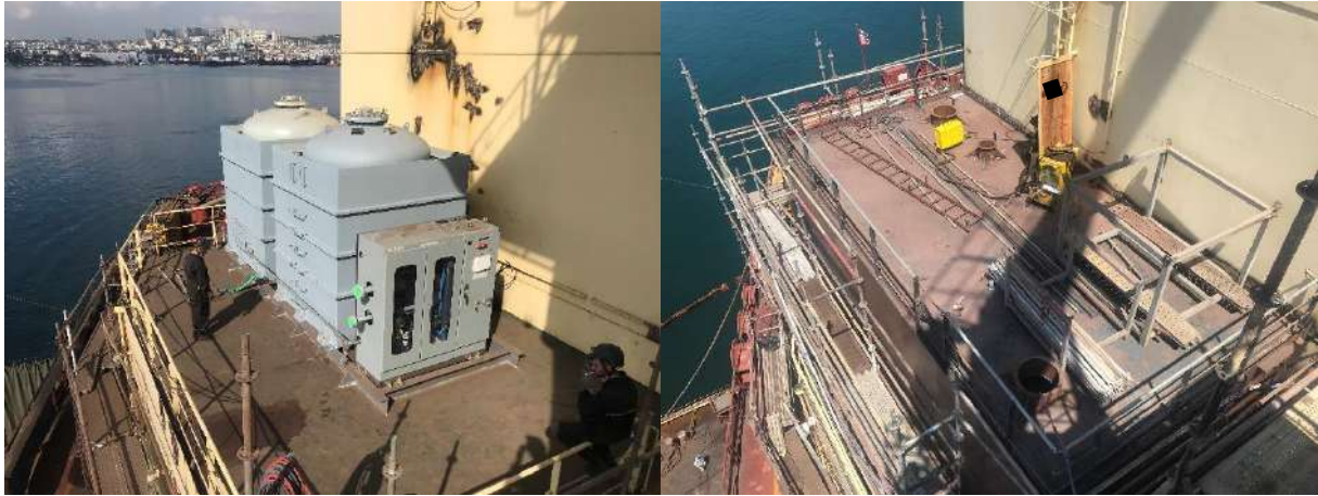
Figure 220 - BWTs Chemical Tank and Deck House Installations
