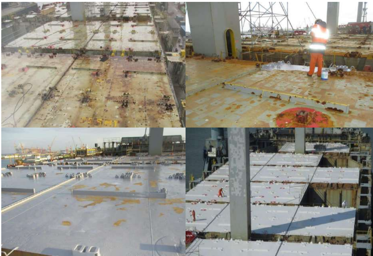
Figure 114 - Waterjetting (500 - 800 bars) and 2 Coat Glassflake Epoxy Application (RA 500M)
