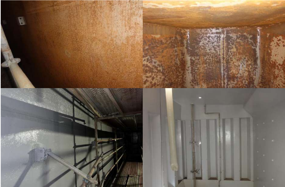
Figure 186 - Chemical Tanker Cargo Tank With Waterjetting (RS 500P + R 500M)
