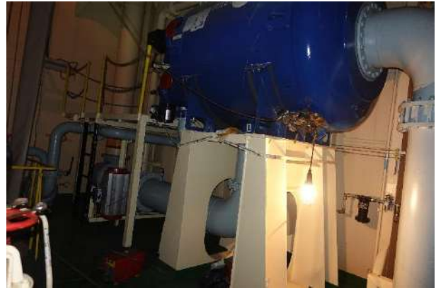
Figure 215 - BWTS Filter Foundation
