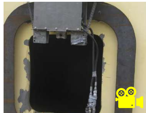
Figure 92 - Cold Cutting with Waterjets (Exproof) on Hull
