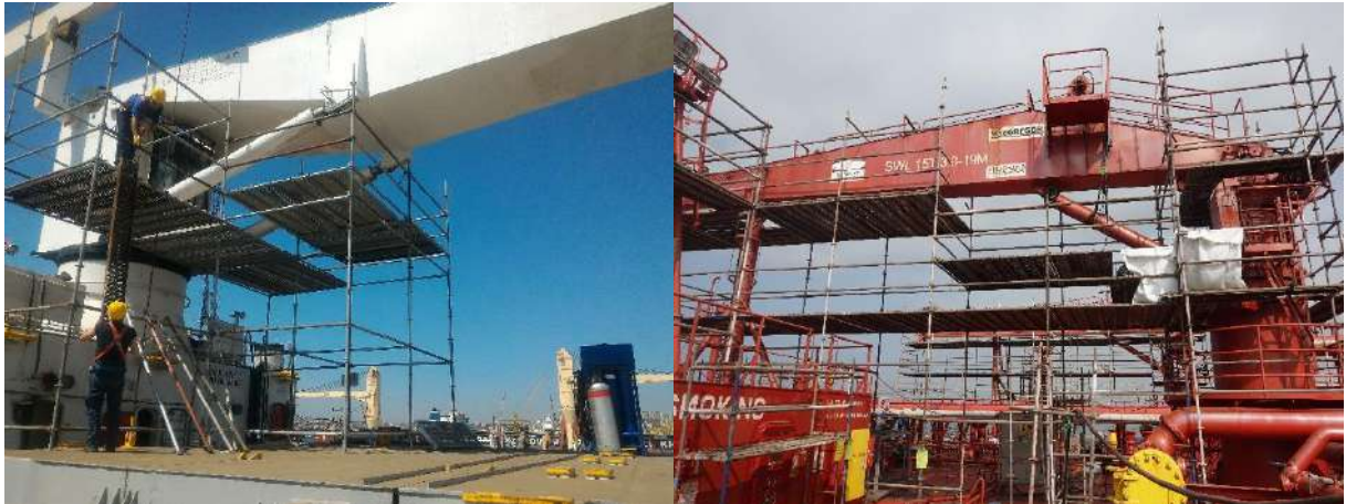
Figure 71 - Crane Hydraulic Piston Repairs with Safe Staging
