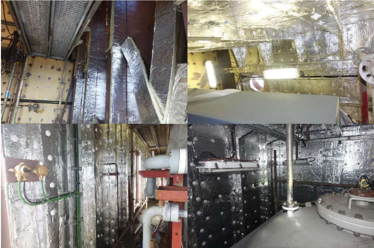
Figure 205 - Insulation for Rooms & Bulkheads
