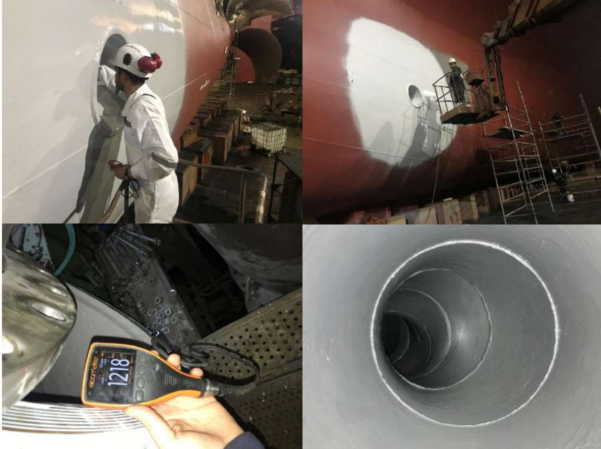
Figure 120 - Scrubber Line and Overboard Protection with Chemco Glassflake Systems
