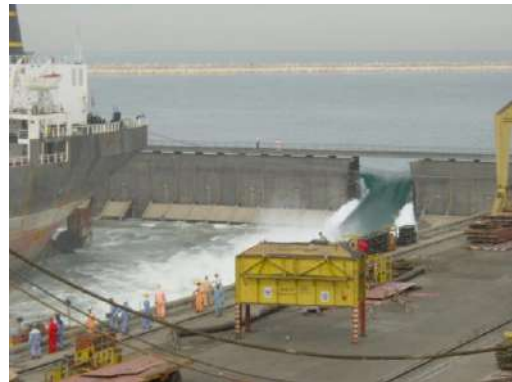
Figure 16 - Failing of Dock Gate
