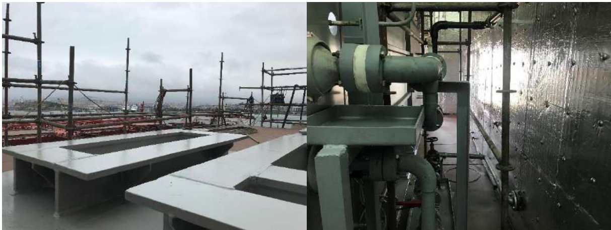
Figure 217 - BWTs Chemical Tank Foundation and Drip Tray Under the Flanges – TK Tuzla Shipyard
