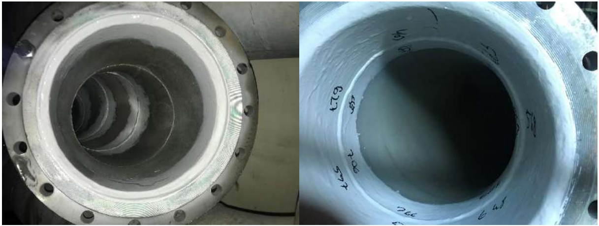
Figure 135 - Repairing (Coating) of Galvanized Pipes with RL 500PF + RA 500M Glassflake
