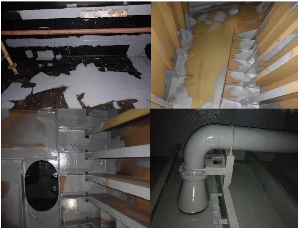
Figure 82 - CAP 1 Final Inspection for Critical Locations in Ballast Tanks
